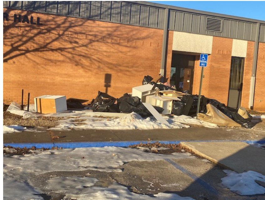
Due to flooding caused by frozen and busted water pipes, carpet and other damaged materials were removed from several classrooms in Tanner Hall.
